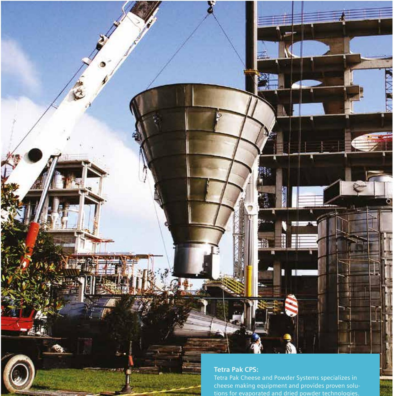
Low-output spray dryer 1,000 per hour (kg/h). Typical plants have an output of 5 MW and a throughput of 5 t/h.
