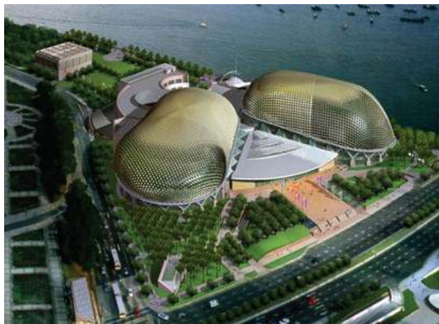
Image from MicroStation, a Bentley Systems product based on Parasolid, courtesy of DP Architects
